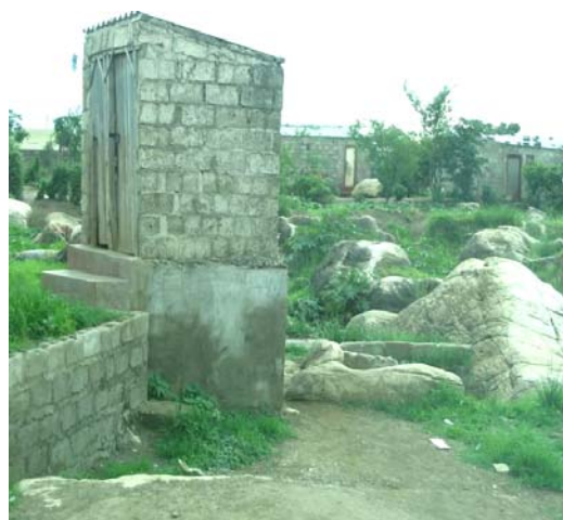
Fig.2: Overhang Latrine in rock out crop
