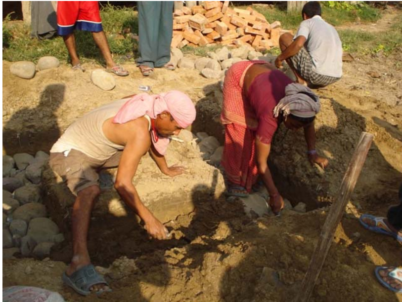
Figure 2: Female LLB, Ms. Khagisara Sapkota busy in latrine construction, Dododhara VDC
